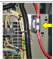
**15A fuse:** lighter fuses are used to protect the control unit, associated wires and the printed circuit against short circuits and amperage peaks.
